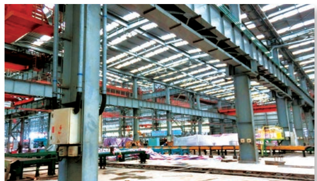
Site staff visited a subcontractor's factory in Guangzhou to monitor the quality and safety aspects
