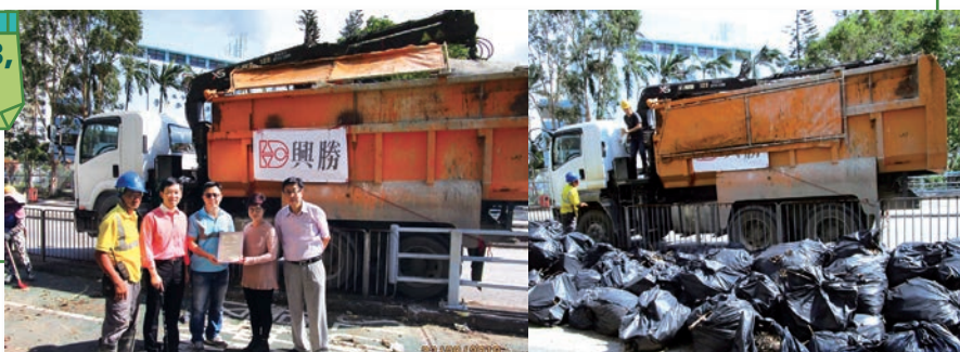
Tai Po clearing of collapsed trees after typhoon
