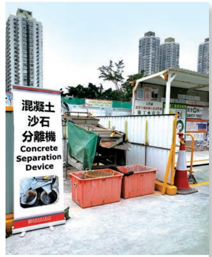
Reuse concrete for backfilling
