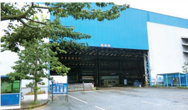
Eastwell Engineering Limited is the subcontractor of construction of Sports Centre, Community Hall and Football Pitches in Area 1 Tai Po of Construction Division
