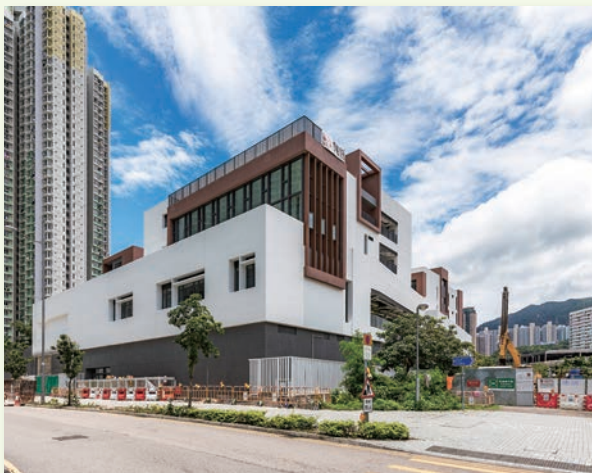
Kai Tak Secondary School Project
