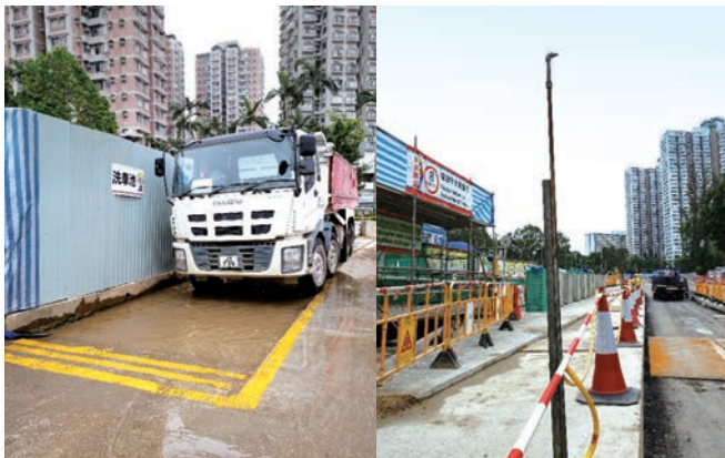
Wheel washing facilities and water spraying for dust control
