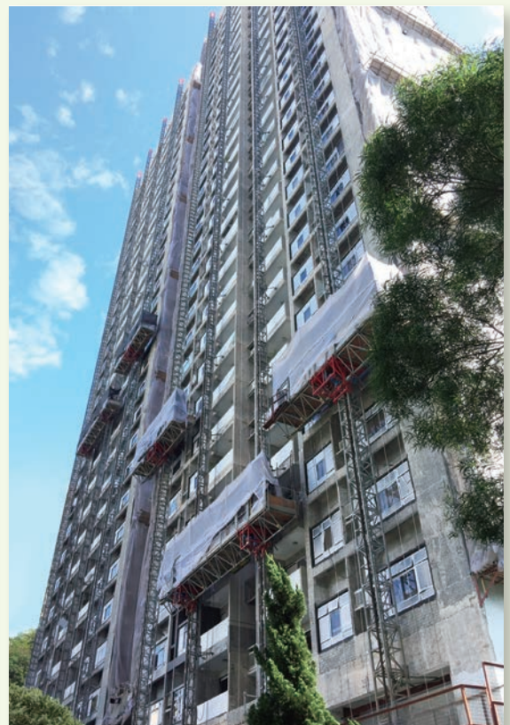
Interior and Renovation Project at Tai Hang Cavendish Height Block 1-7
