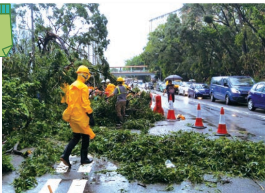
Sheung Shui clearing of collapsed trees after typhoon
