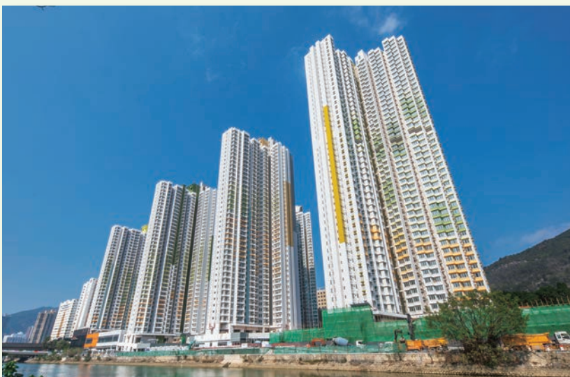
Construction Project at Sha Tin Shek Mun Estate Phase 2
